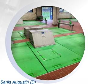
12 × 60 m² disk filters flocculation filtration 4'540 m³/h, Total P < 0.65 mg/l
